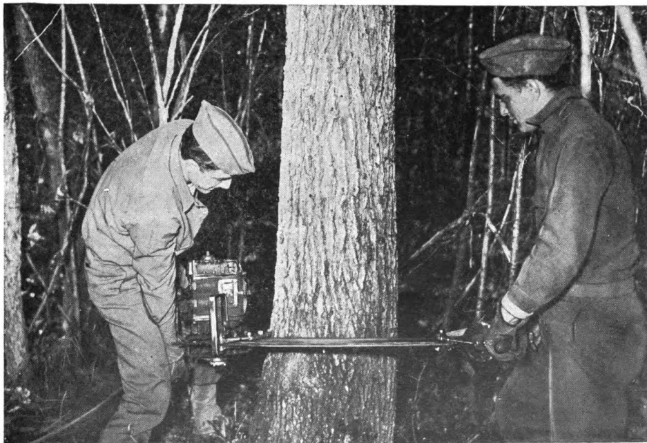
Figure 44. Pneumatic chain saw used in tree clearing.
